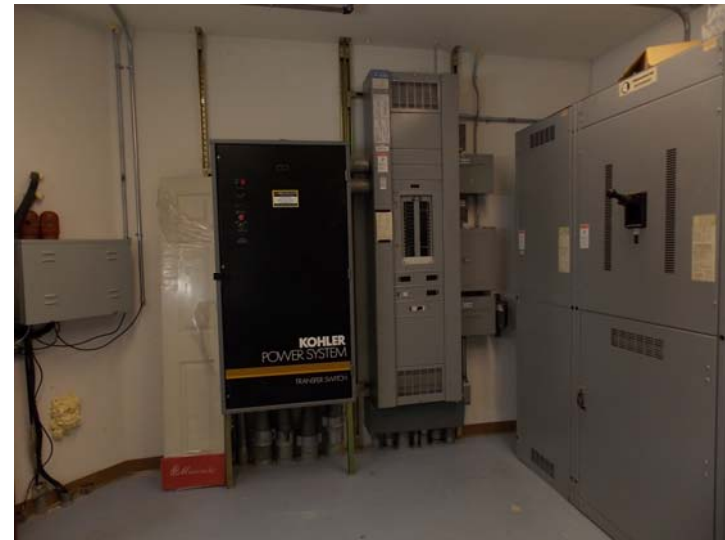
This is the transfer switch for the emergency generator.
