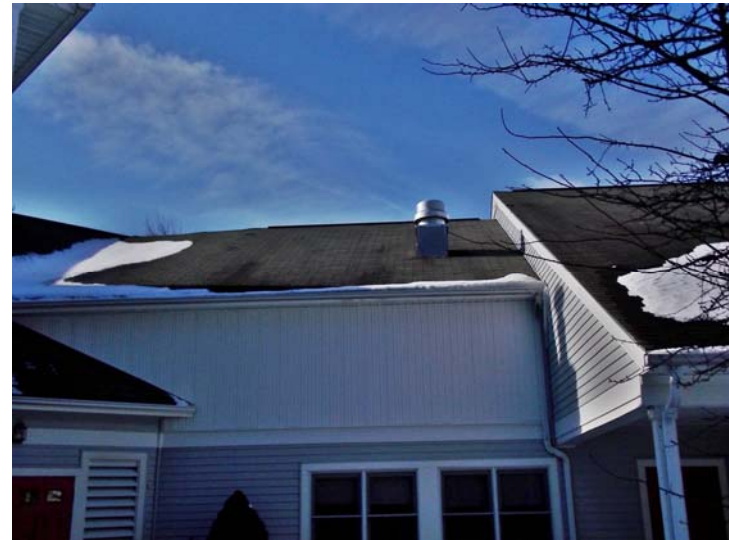
The building is clad with vinyl siding, And has asphalt shingle roofing.
