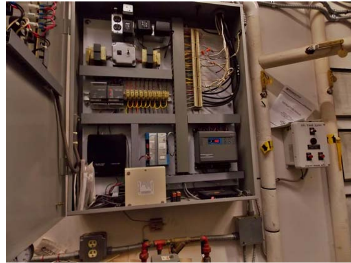
The boiler plant is governed by this computerized controller.
