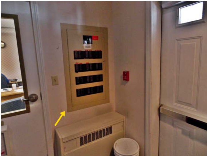
This fire alarm control panel (FACP) governs the common area alarm and detection devices.
