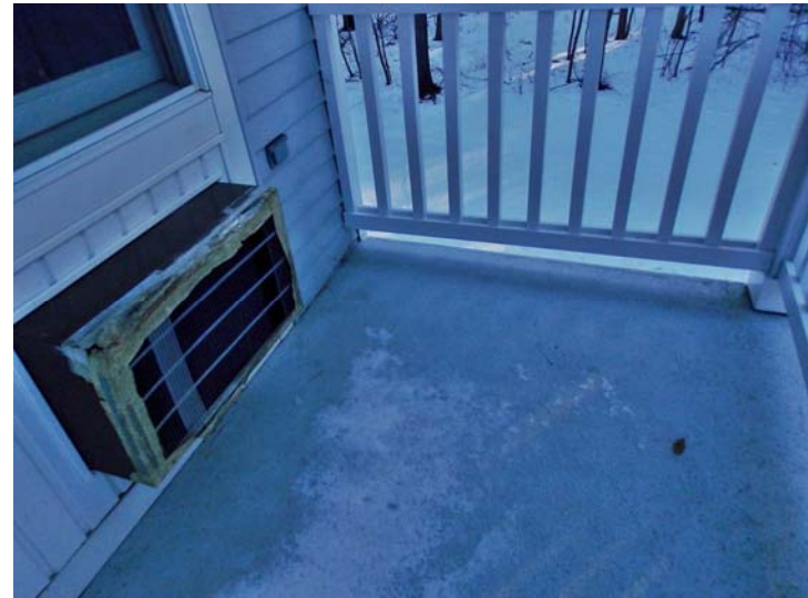
Private balconies have concrete decks and wood railing.
