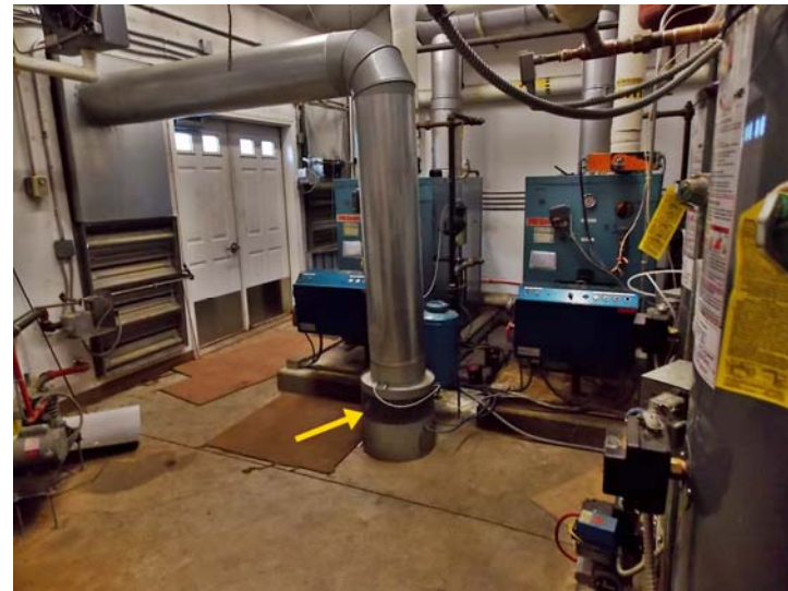
This fan, which is controlled by the burners' circuit, provides fresh air for combustion.
