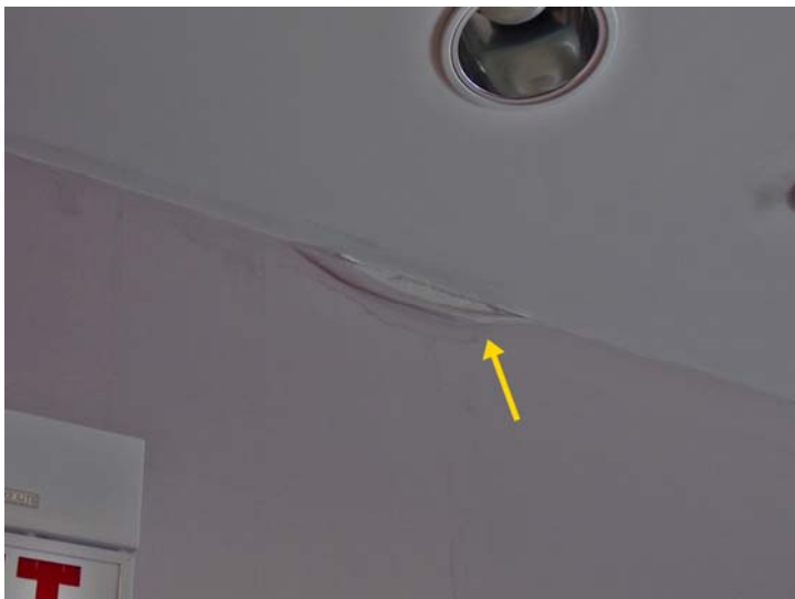
A close-up of peeling paint, the result of water infiltration from a roof leak.
