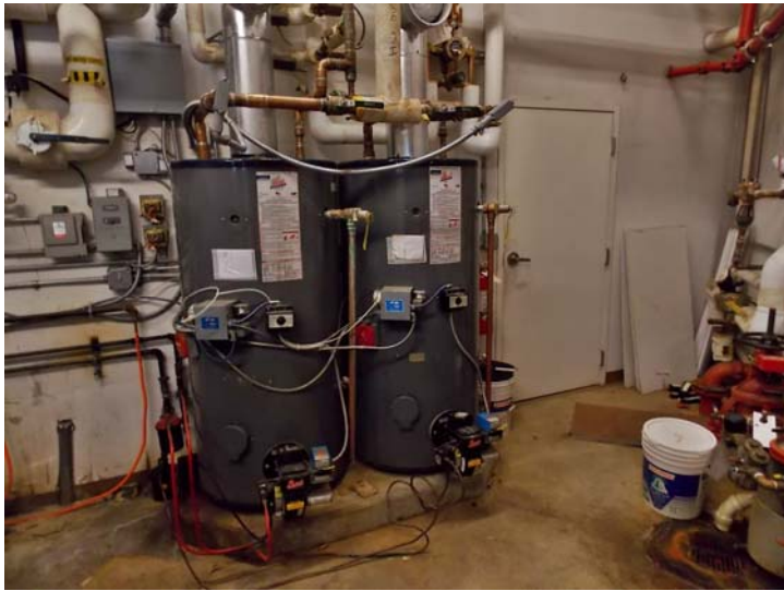
Domestic hot water is generated by and stored in this pair of oil-fired DHW tanks.
