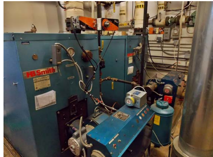
The boiler plant consists of this pair of oil-fired hydronic boilers.
