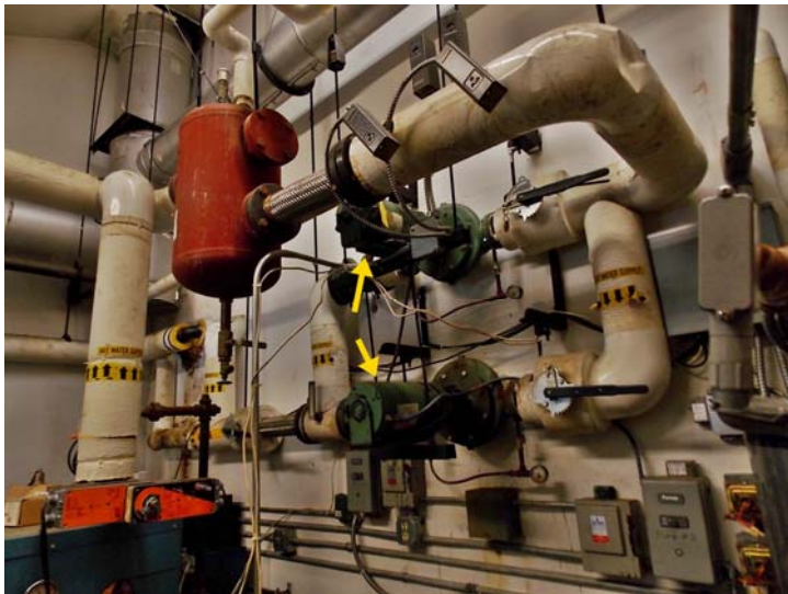
This pair of hydronic heat circulating pumps serves the entire facility.
