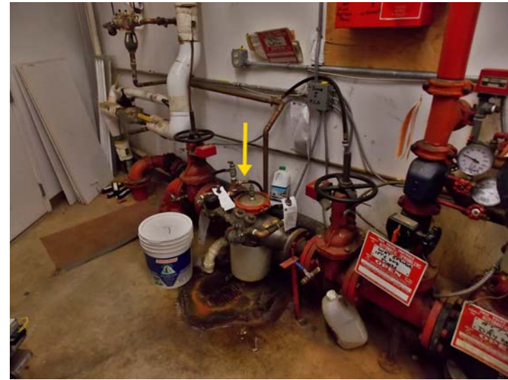
The fire sprinkler system includes a backflow preventer (arrow).
