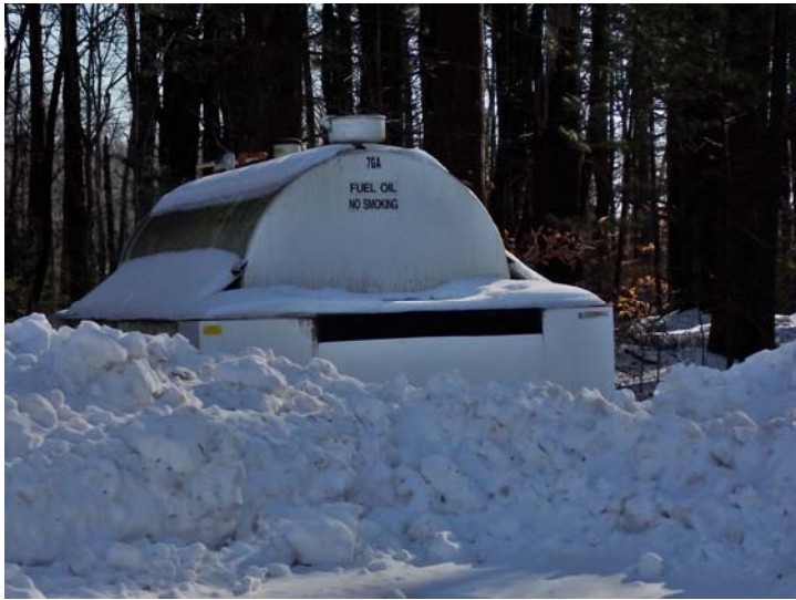
Fuel oil is stored in an above-ground tank.
