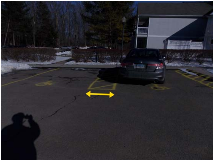
This access aisle needs to be re-stripped to the compliant width of 60 inches.
